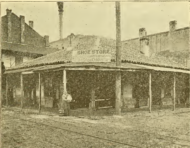
Spanish Tile Roof House at the Corner of Chartres and Dumaine Streets, recently demolished.
